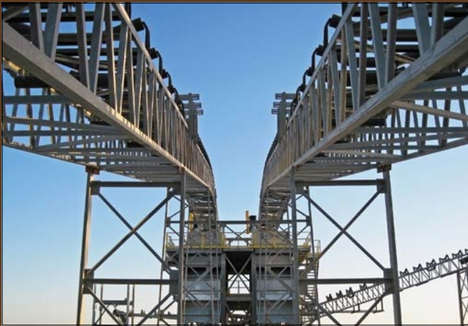
Abu Dhabi Aggregate Recycling Plant Abu Dhabi, United Arab Emirates
