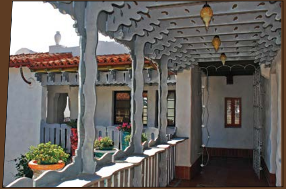
El Andaluz Commercial Offices & Residences Santa Barbara, California
