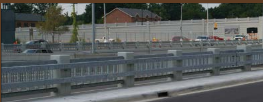
M-102 Bridge Rail Reconstruction Detroit, Michigan
