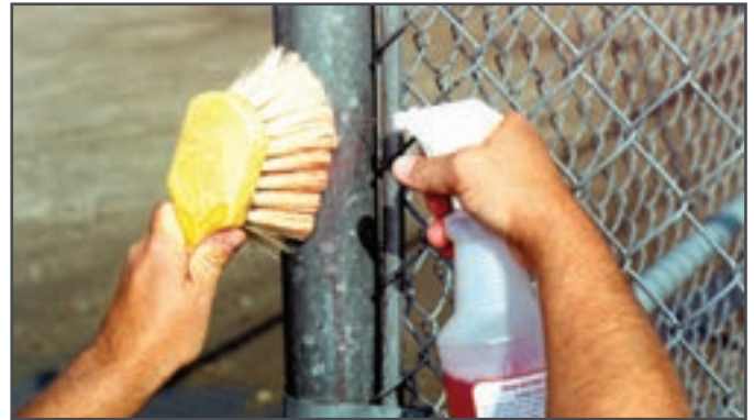
Cleaning galvanized steel
