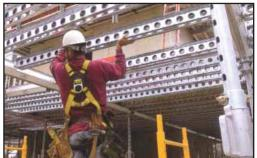
In 2007, EFCO, a manufacturer of systems for concrete construction, began marketing a newly developed Handset Shoring System for cycling large deck panel systems from floor-to-floor by crane. The innovative system and lightweight components of this project are designed so one person can erect the shoring system without the assistance of an entire crew.
